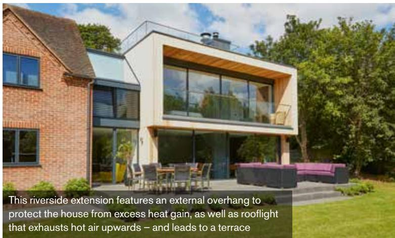
This riverside extension features an external overhang to protect the house from excess heat gain, as well as rooflight that exhausts hot air upwards – and leads to a terrace
